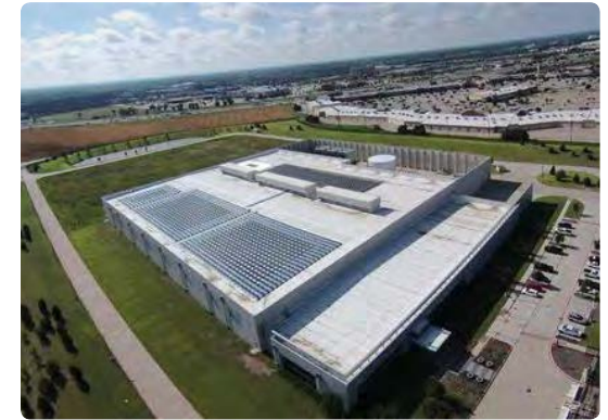
Cisco's Allen, Texas, Data Center Solar Project
